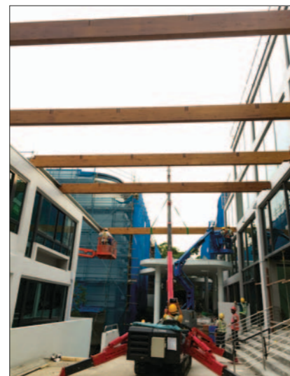
Nanyang Technological University Hall of Residence 5 under construction: The new canopy features the first European Spruce glulam beam imported to Singapore with local regulatory approval.
