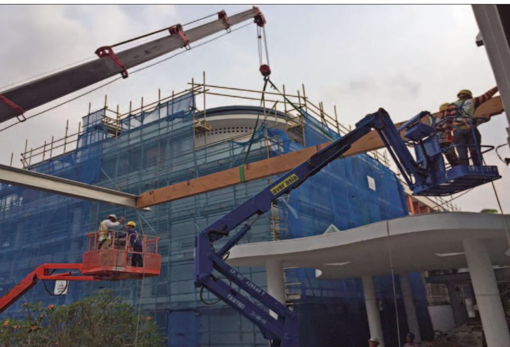
Nanyang Technological University Hall of Residence 5 under construction: The new canopy features the first European Spruce glulam beam imported to Singapore with local regulatory approval.
